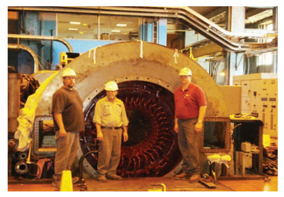
Onsite turbine generator rewinds (22 MW / 13.8 kV / 3,600 RPM)
