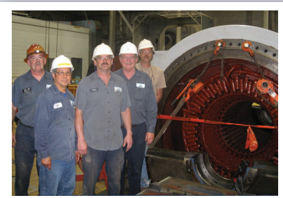
IPS Field service technicians work on a 44 MW GE hydrogen-cooled generator.
