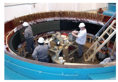
Onsite hydroelectric generator rewind (10 MW / 6.9 kV / 171 RPM)
